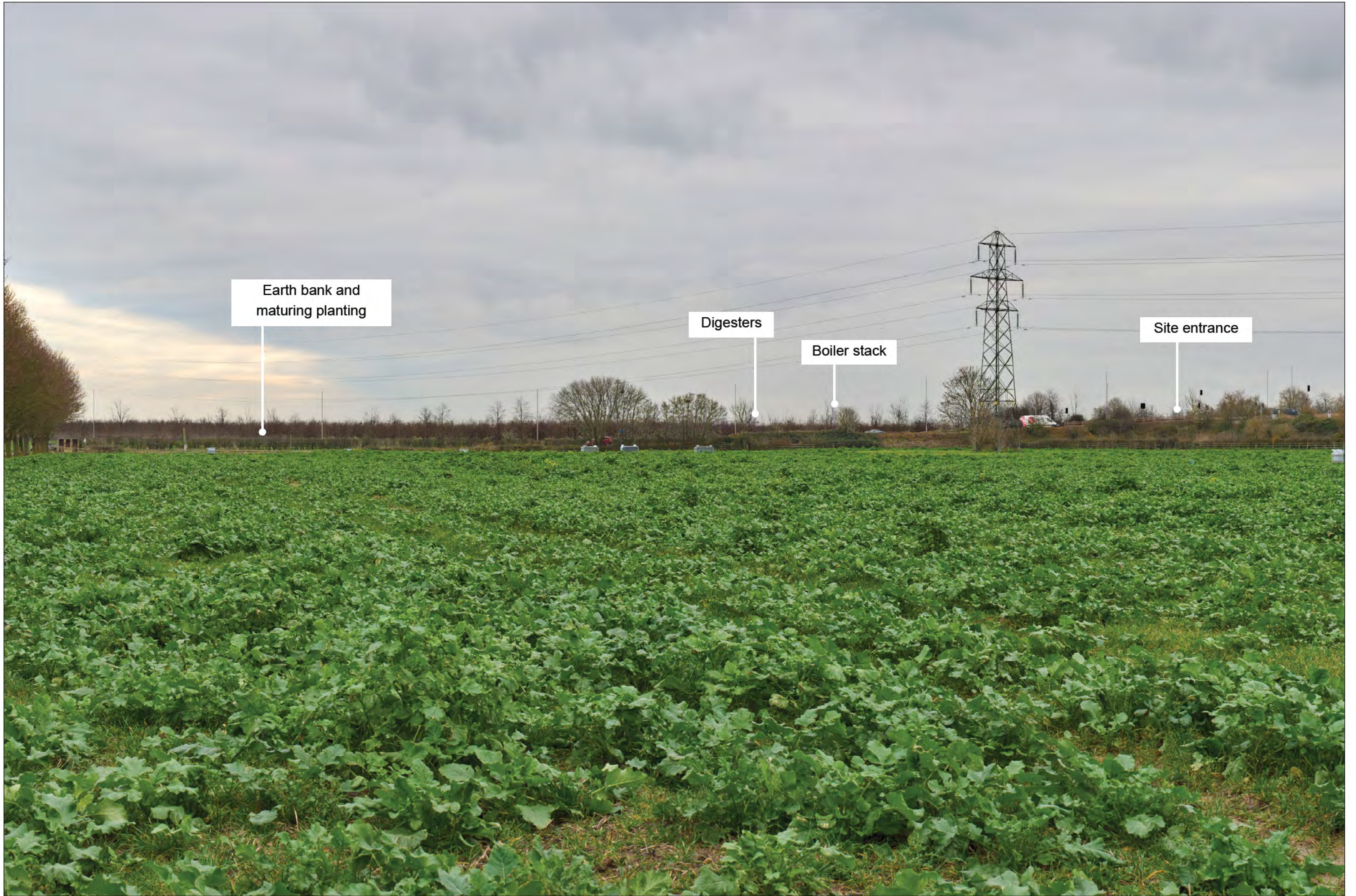
Photomontage 2: Year 15 in operation (planar projection, field of view 39.6 degrees x 18 degrees, to be viewed at A3) Cambridge Waste Water Treatment Relocation Project: Photomontages
